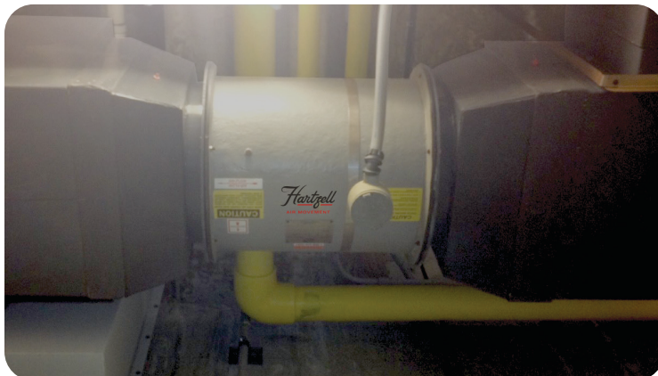
Series 28 Fiberglass Direct Drive Duct Fan in Caustic Soda Room at a Water Treatment Plant
