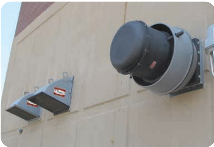
Series 88 Fiberglass Exhauster with Electrostatic Grounding and Hoods
