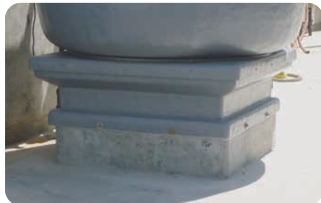
Series 88 Fiberglass Exhauster with Custom FRP Base
