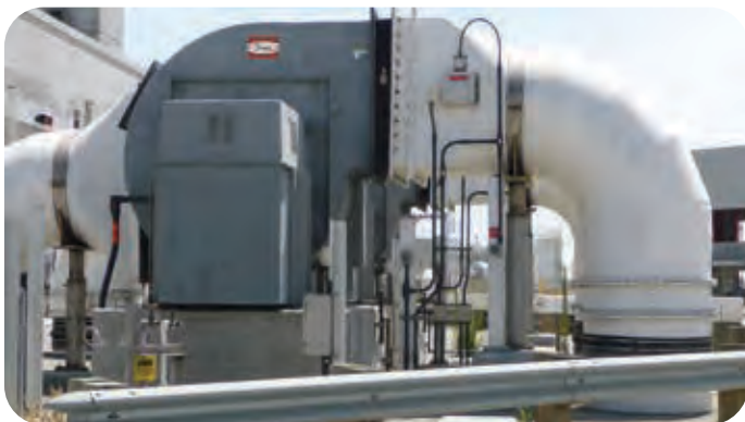
Series 41 Fiberglass Backward Curved Centrifugal Fan
