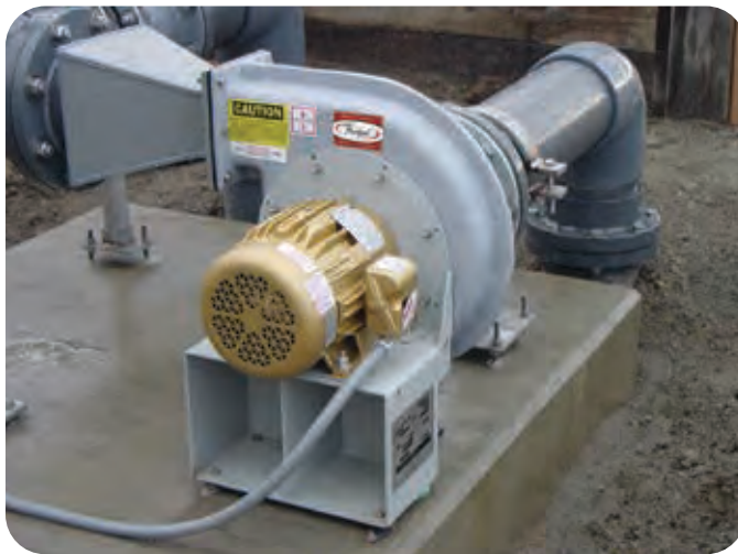
Series 42 Fiberglass Pressure Blower at a Wastewater Treatment Plant
